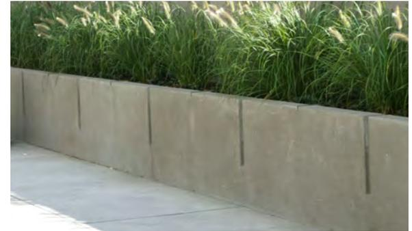
Cast-in-place concrete retaining wall with integrated planters
