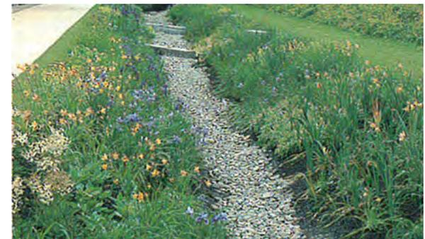
Stormwater swale with crushed rock channel and check dams
