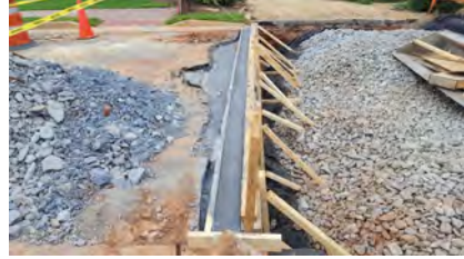
Concrete Cut Off Wall
