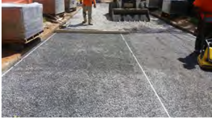
Base Stone Layer and Compaction
