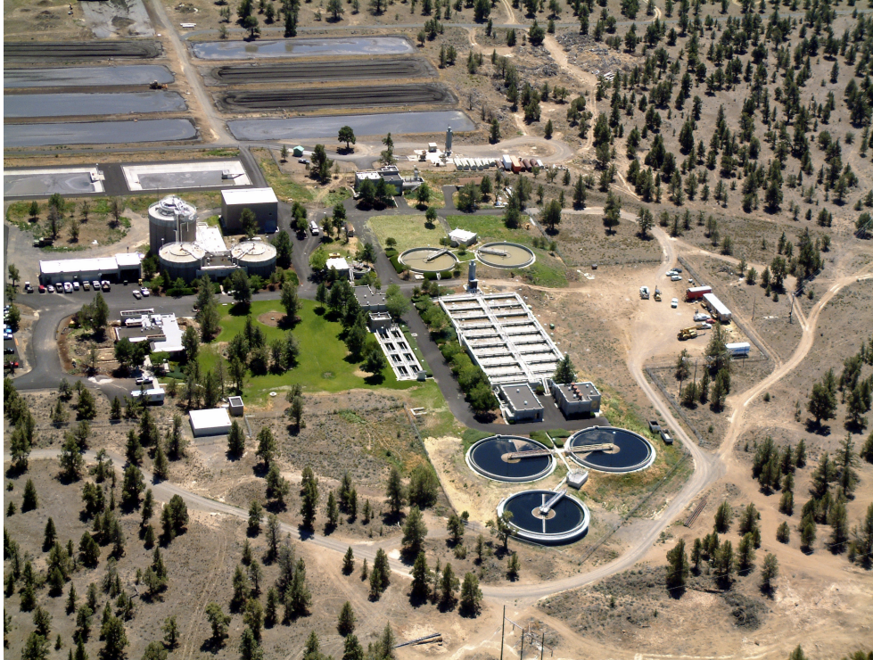
Aerial Photo of the Water Reclamation Treatment Plant
