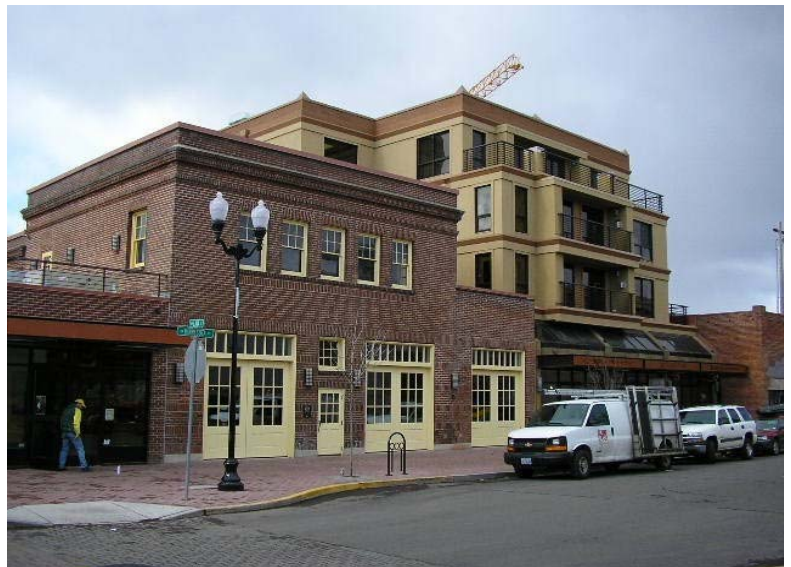
Old Fire Hall (redeveloped in 2006)
