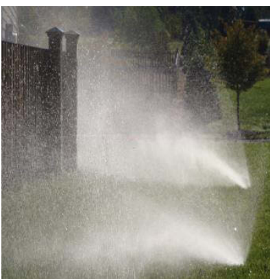
Operating under too much pressure can cause misting, fogging, overspray, and uneven coverage. Courtesy of the Irrigation Association.
