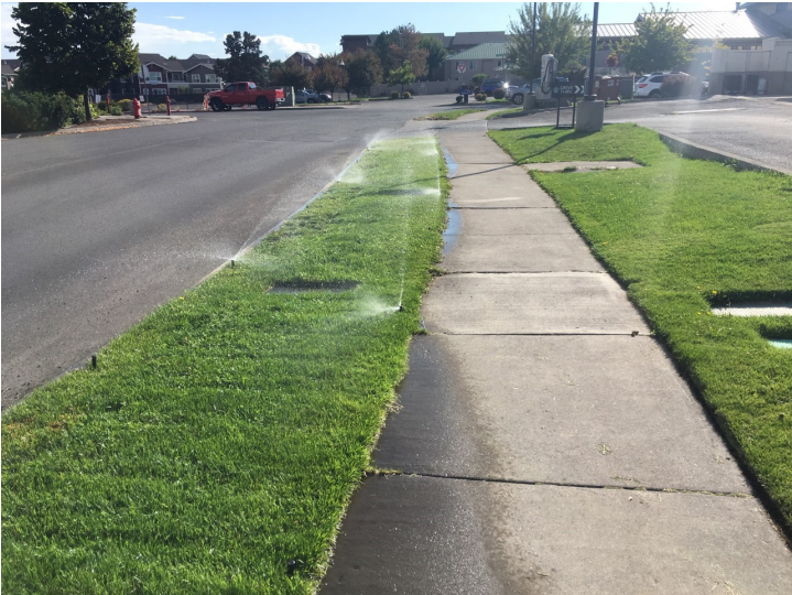
AFTER: The contractor shut flow to every other sprinkler, creating a proportionate area in which strip spray nozzles are a much better fit.
