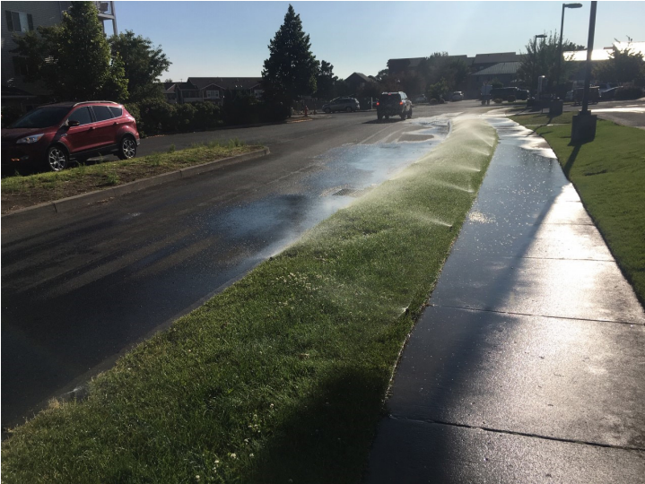
BEFORE: High pressure, obstructed sprinklers, disproportionate nozzles and improper scheduling all contribute to water waste at this site.
