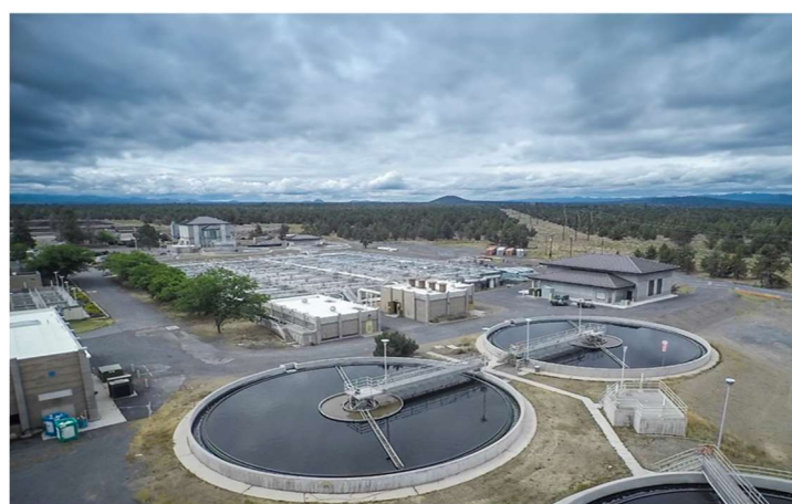
Water Reclamation Facility – looking SW towards the City. Secondary clarifiers in foreground.
