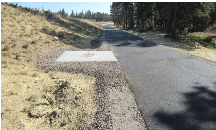
SW Sewer Basin Phase 2A
