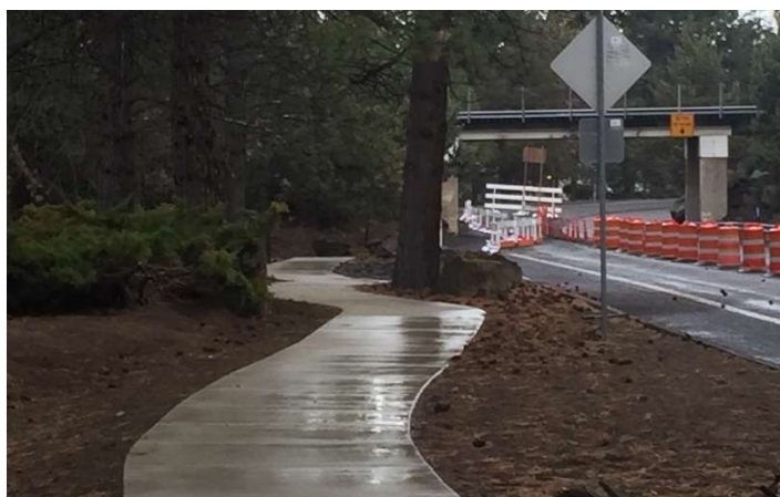
New Brosterhous sidewalk west of railroad bridge
