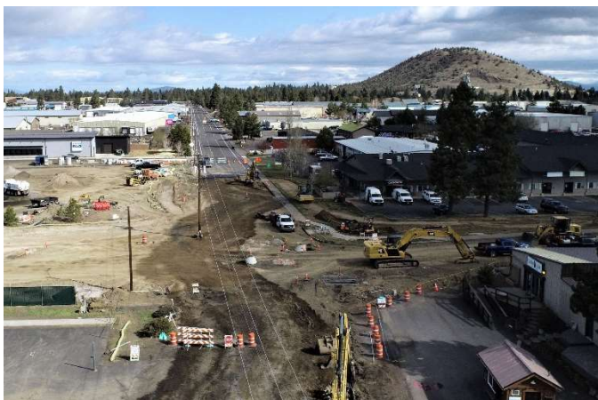
Ninth Street and Wilson Avenue construction
