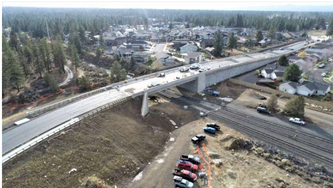
Murphy Bridge over BNSF Railroad
