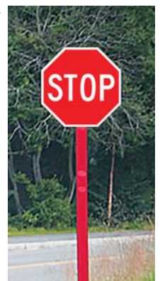
Example of reflective strip on sign post.
