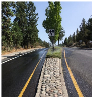
Irrigation overspray and runoff due to overhead irrigation in a parkway median landscape.
