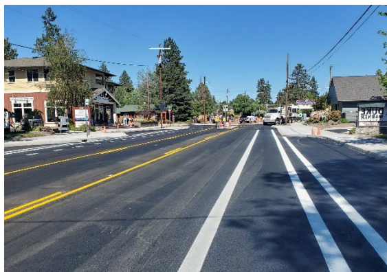
Segment 2B roadway opens. Construction begins on segments 2C and 3.
