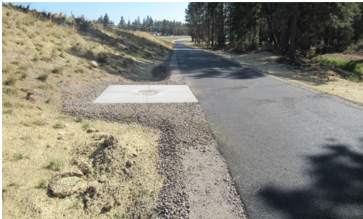
SW Sewer Basin Phase 2A
