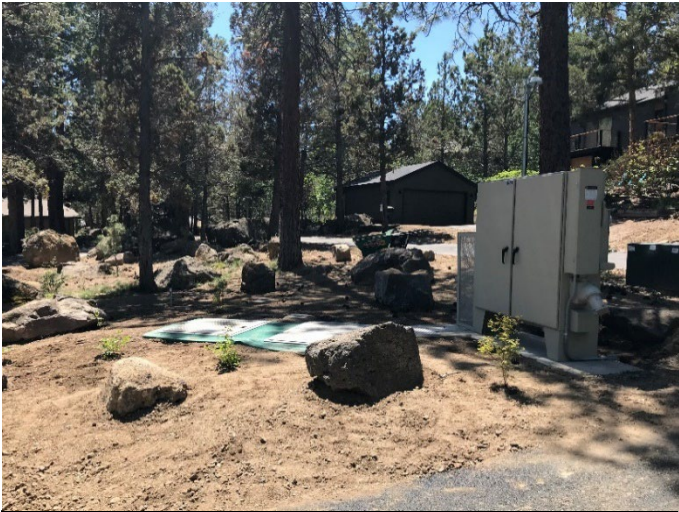
Completed Rimrock Pump Station #2
