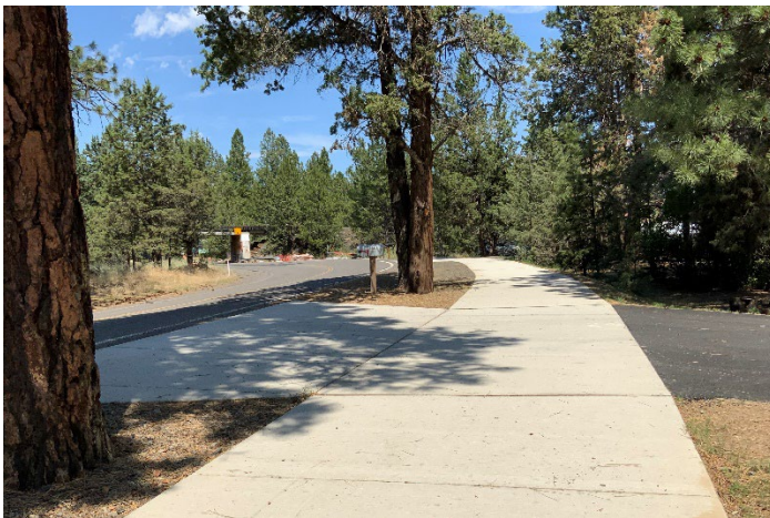
New Brosterhous sidewalk east of the railroad bridge
