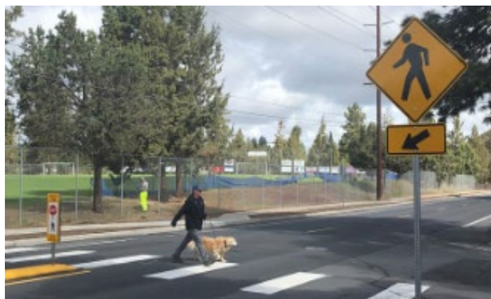
Crosswalk Safety Project at the intersection of 15 th Street and Virginia Road (Completed 2020)
