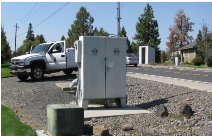
Camden Pump Station to be decommissioned during construction of Phase IV
