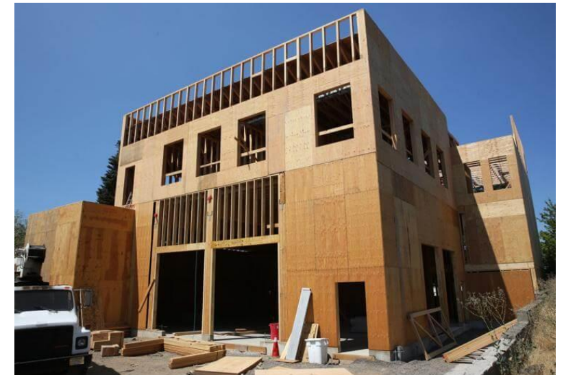
DVAA & Imagine Stone Works Office, 221 NE Hawthorne Ave. CofO issued August 2022
