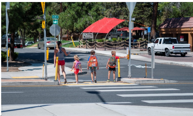
Third Street safety island and crosswalk flashing beacon (photo credit: Craig Powell Photography)
