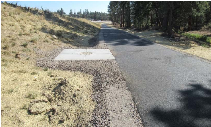
SW Sewer Basin Phase 2A
