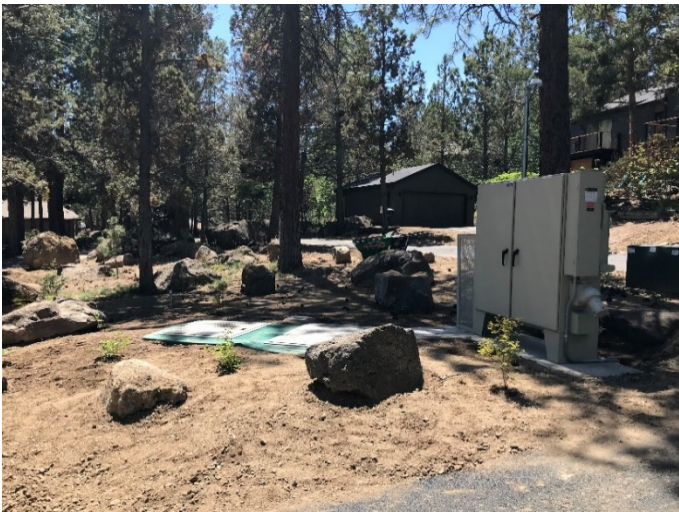
Completed Rimrock Pump Station #2
