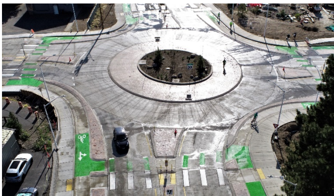
Ninth Street and Wilson Avenue roundabout
