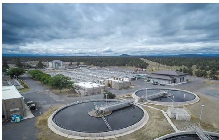
Water Reclamation Facility – looking SW towards the City. Secondary clarifiers in foreground.
