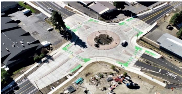
Improvements at Wilson Avenue and 9th Street
