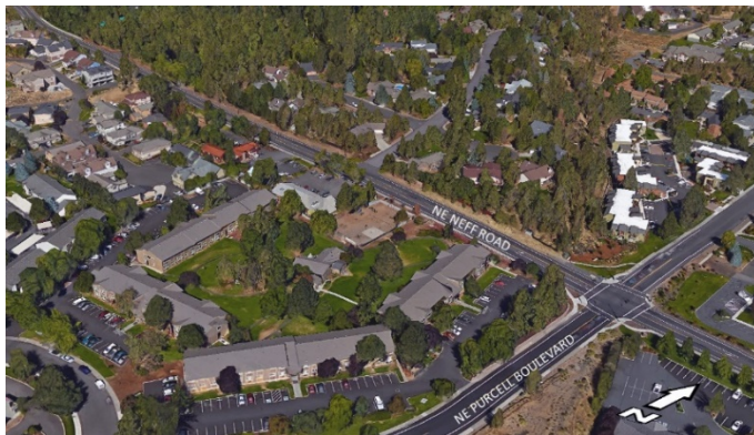
Neff & Purcell Intersection
