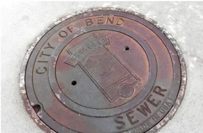
City of Bend standard collection system manhole lid.
