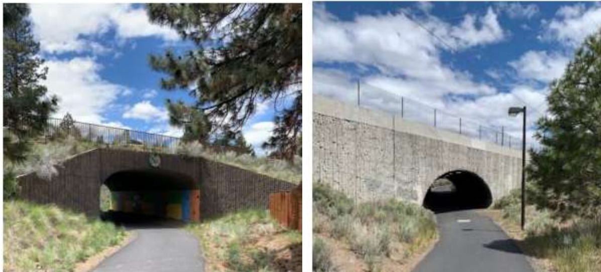
Figure 51 - Image trail under crossings that eliminate the conflicts of at-grade crossings to improve safety and travel time for all users
