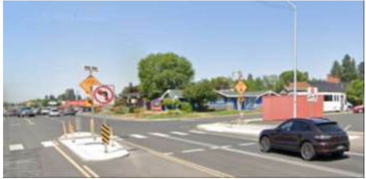
Figure 35 - Enhanced Crossing with Rectangular Rapid Flashing beacon
