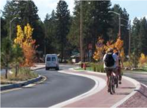
Figure 22 - Raised Bike Lane
