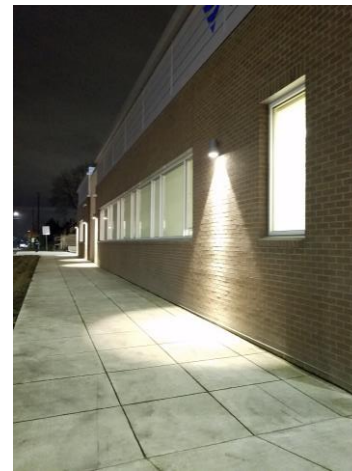
Desired lighting outcomes of a cylinder downlight – a strong directed pool of light.
