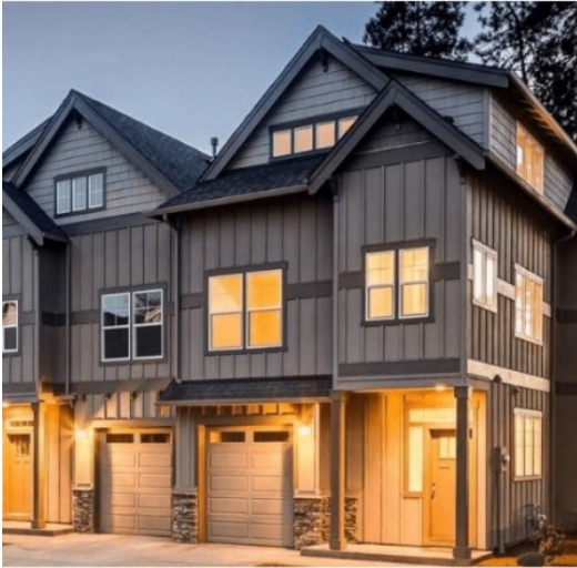
Townhomes on Reed Market Rd, Bend
