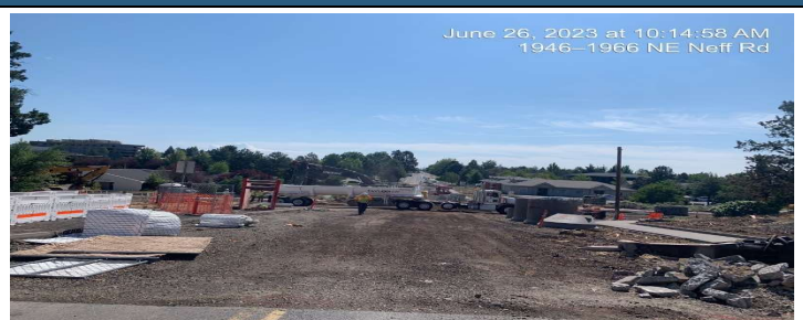
Installation of sewer pipe within the intersection
