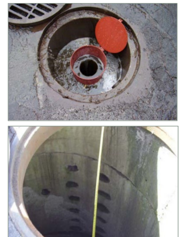
Figure 1-1. Drill hole (top); drywell interior (bottom)
