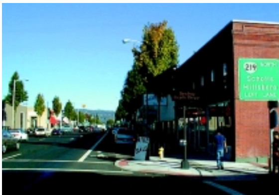
Completed curb extension and bike lane.
