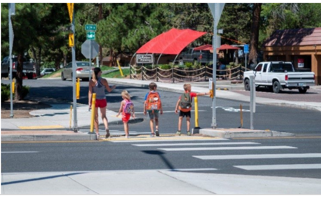
Third street safety island and crosswalk flashing beacon (photo credit: Craig Powell Photography)
