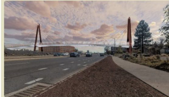
Option 1 - Cable Stayed-Two Towers
