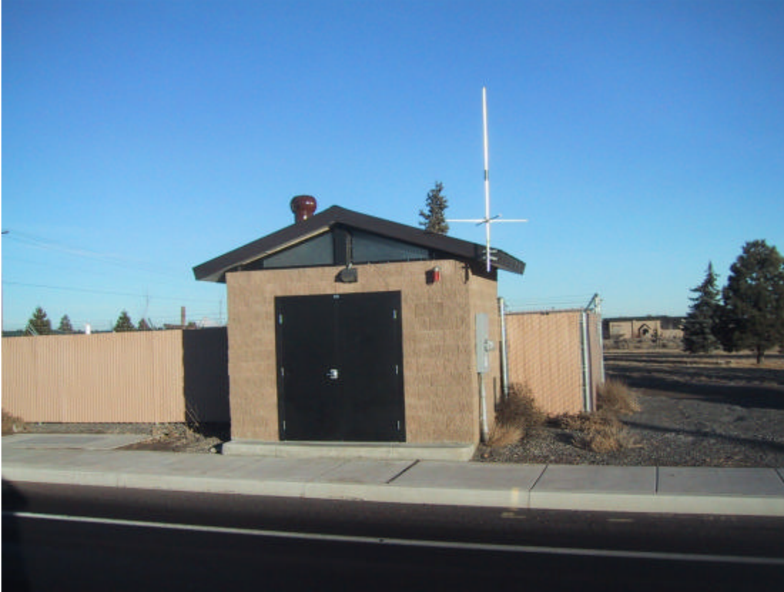
Avion/Bend Interconnect – Chlorine Injection Building, Valve is in Vault
