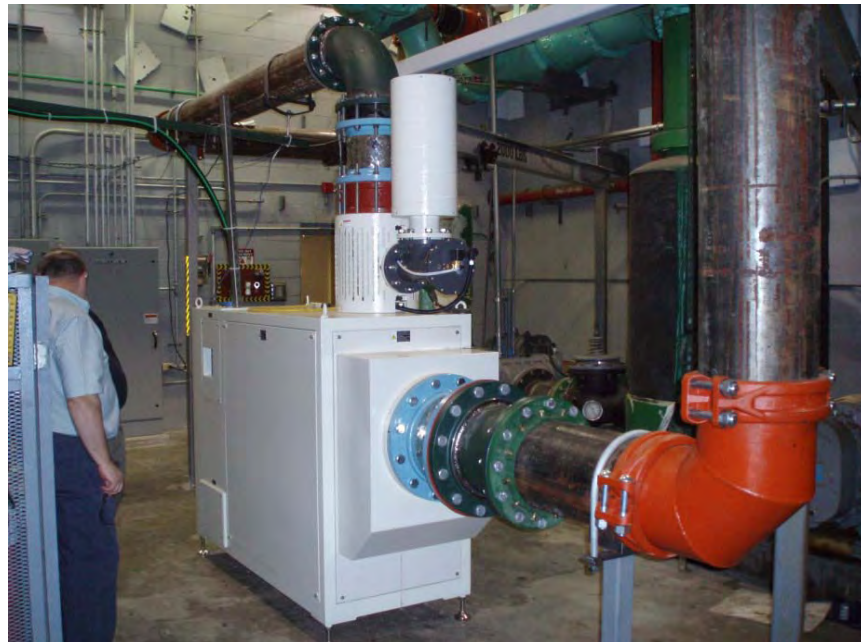
Models NX75 to NX150 Enclosure and Installation Layout
