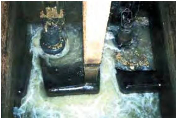
5- Self-cleaning action occurs throughout the prerotation cycle, resulting in a clean wet-well every time the prerotation cycle occurs.
