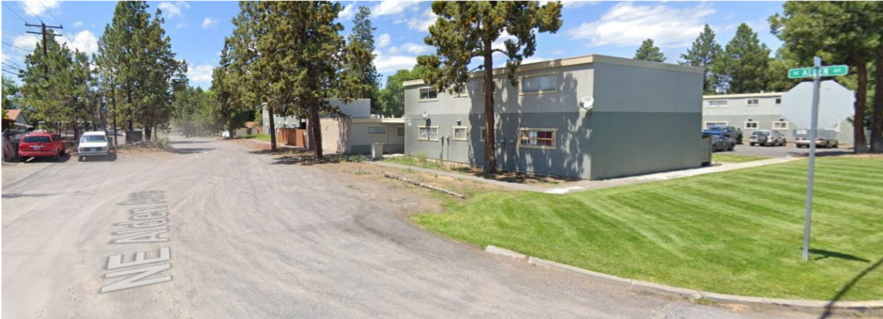
Alden Gravel Street – not accessible
