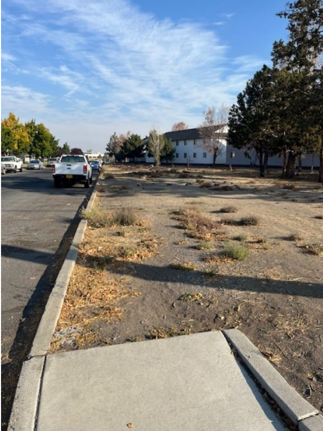
Watt Way Missing Sidewalk
