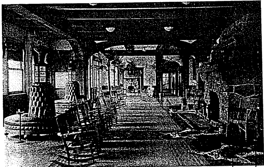
Bend's Pilot Butte Inn is scheduled for demolition next week. In its 56 years it has hosted such guests as Eleanor Roosevelt and Herbert Hoover, as well as such local functions as banquets, art shows and weddings. Since its early years, both the exterior (above) and lobby (left) have been changed by wear and remodeling.
