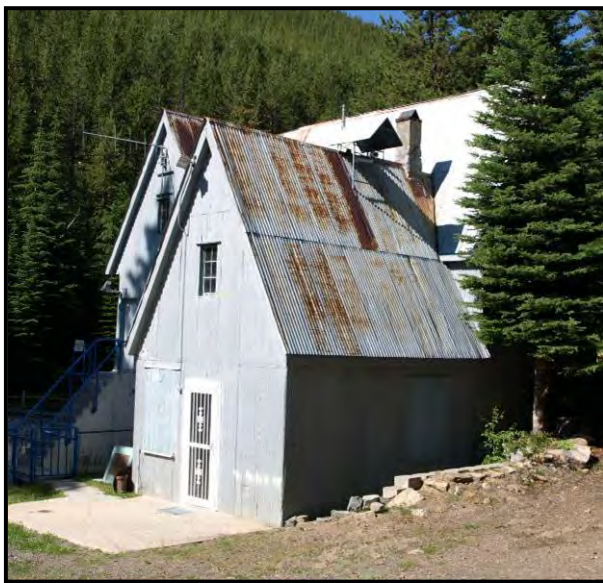
Figure 7.16. North elevation, showing shortened masonry chimney.
