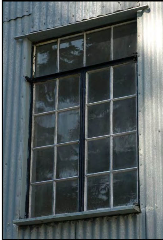
Figure 7.15. Original steel sash casement window with 4-light transom.
