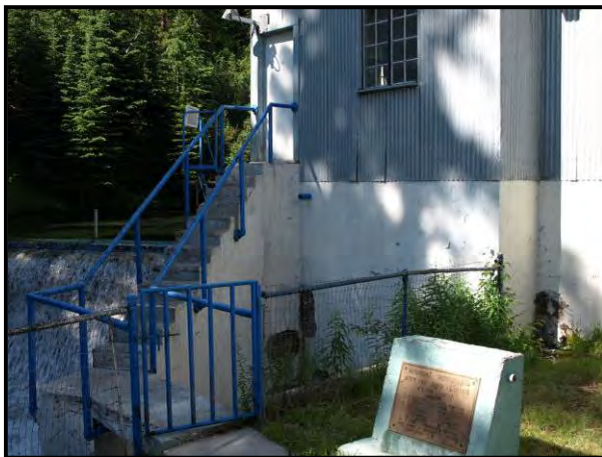
Figure 7.19. East elevation, outside stairs to screen chambers.
