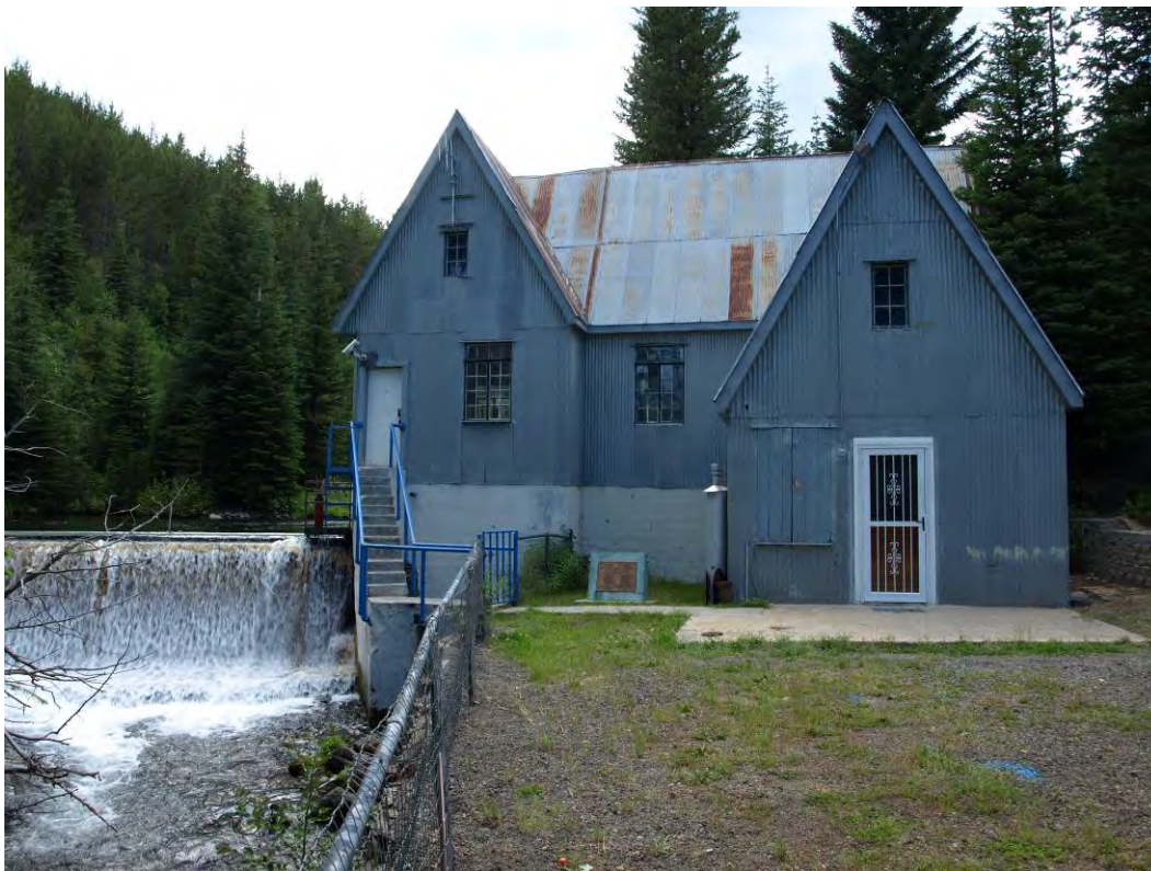
Figure 7.14. Current condition of the east or entry elevation, intake building.
