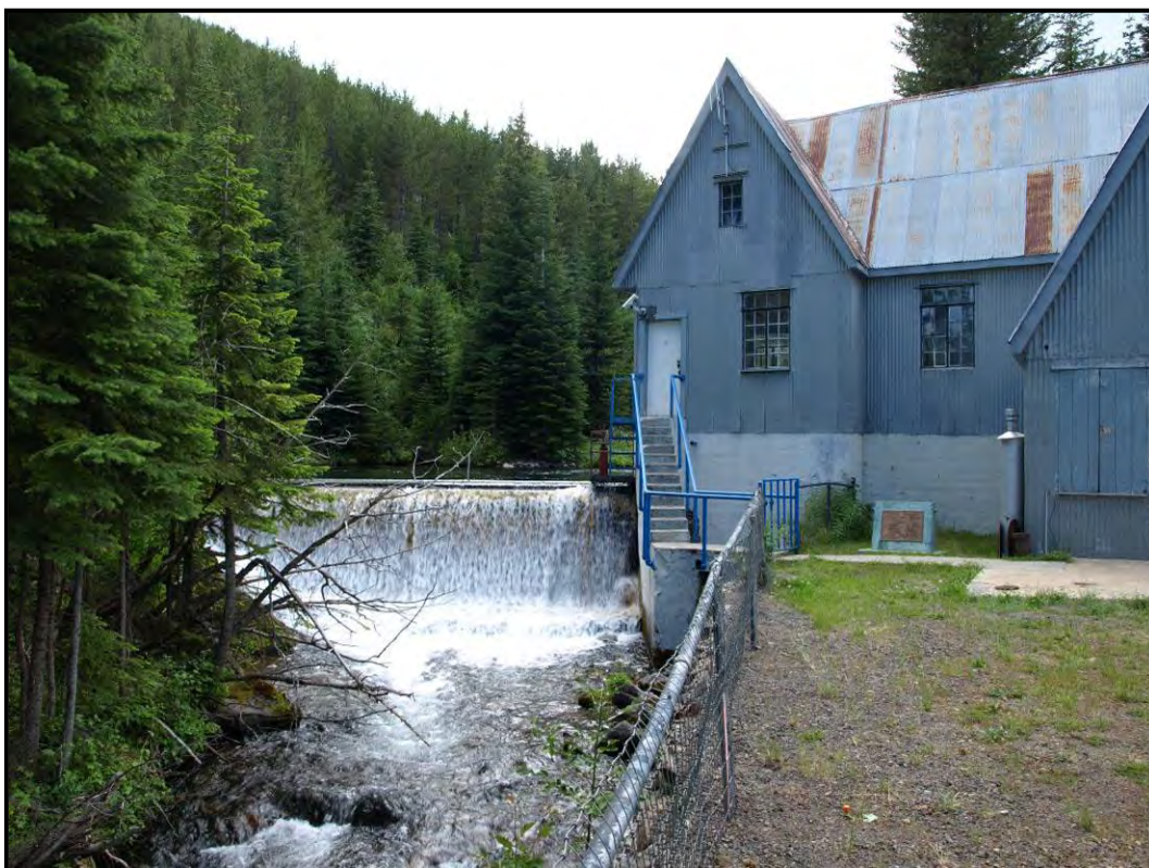
Figure 7.2. Dam and intake building, looking west.
