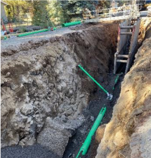
Eight-inch sewer and service lateral
