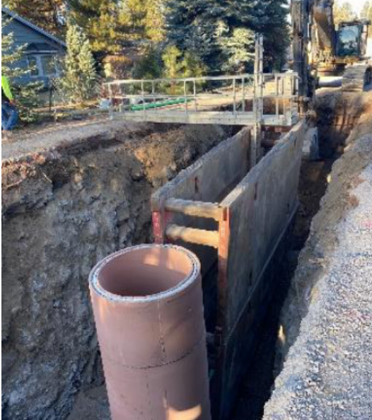
Manhole and pipe install
