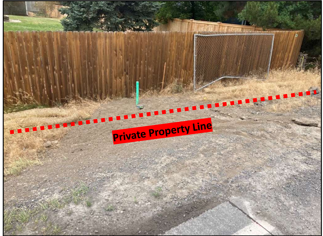
Gravity Sewer Service Lateral
