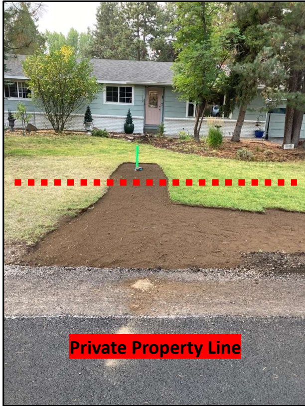
Gravity Sewer Service Lateral
