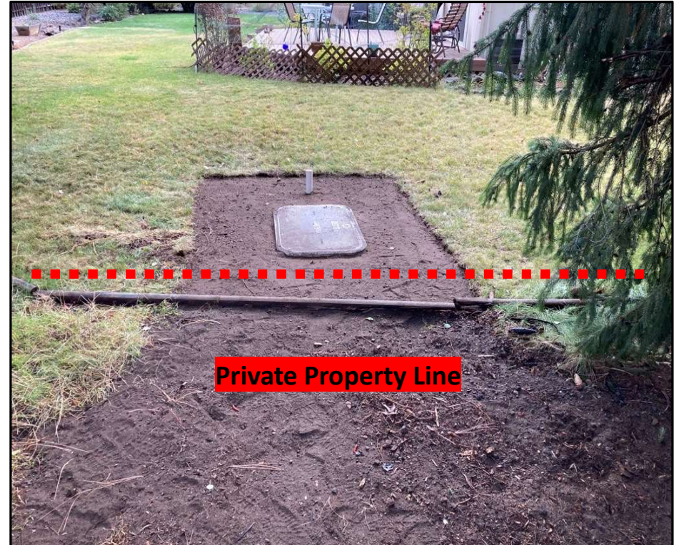
Pressure Sewer Service Lateral
