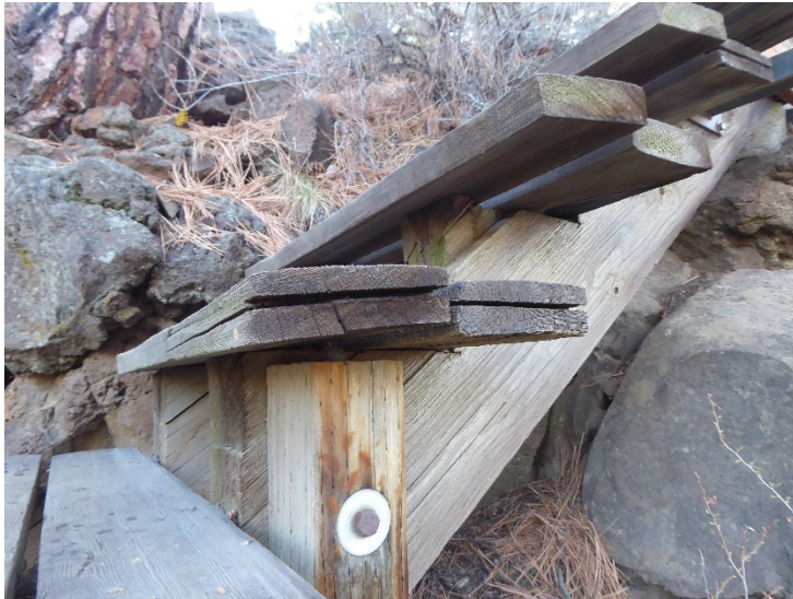
Photograph 5: Checks and splits in treads.
