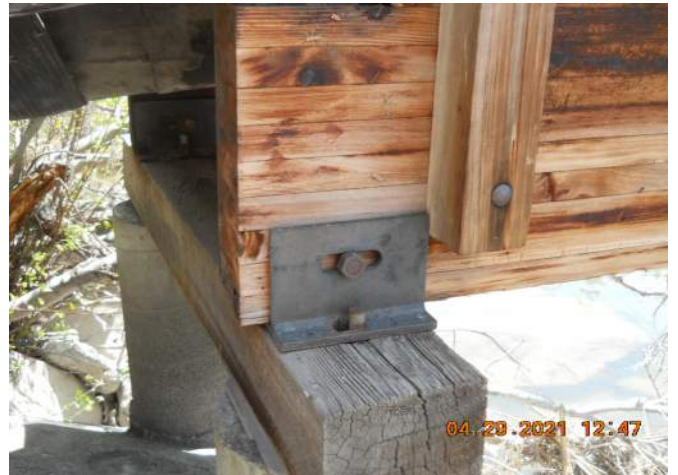
Bent 6 North Bearing Plate Missing Nut
