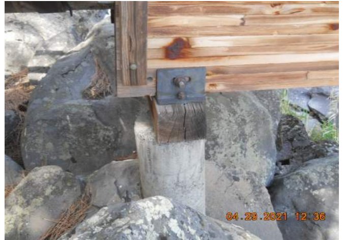
Full Depth Split in Bent 3 Cap
