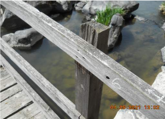
Top of Railpost Section Loss
