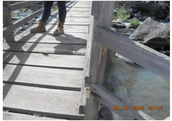
Railing Notched into Railposts
