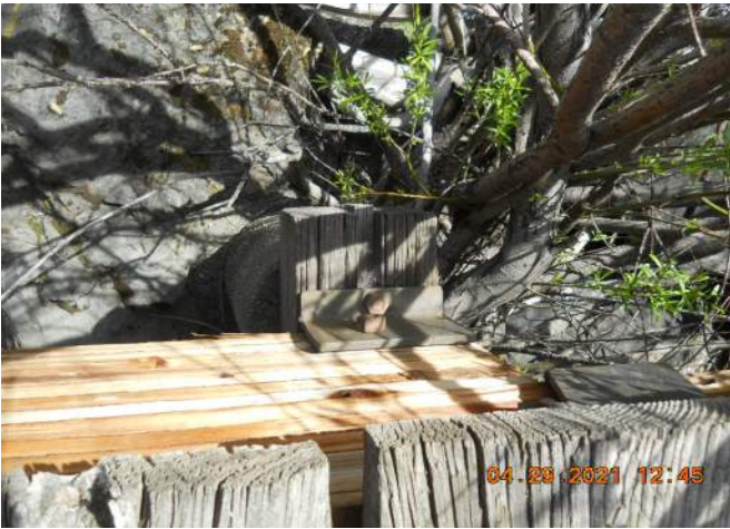
Bent 5 Cap Split at South End
