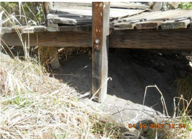
North Post Not Fully Bearing at Bent 7A
