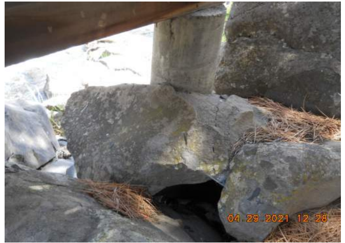
Bent 3 Concrete Column on Rock w/Void Underneath
