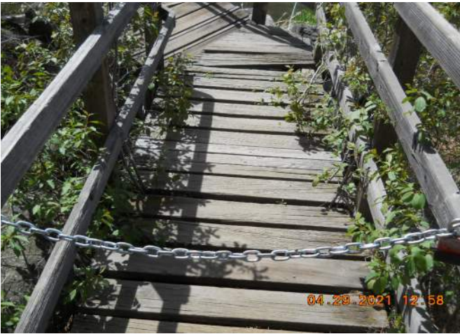
Missing Decking at Span 8 West End
