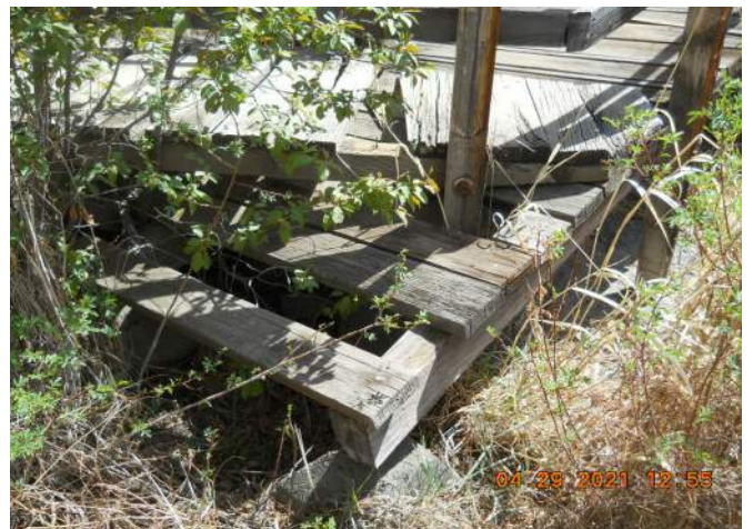
Overlapping Decking at Span 7 to Span 8
