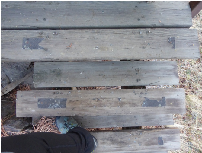
Photograph 8: Stair treads varying widths.
