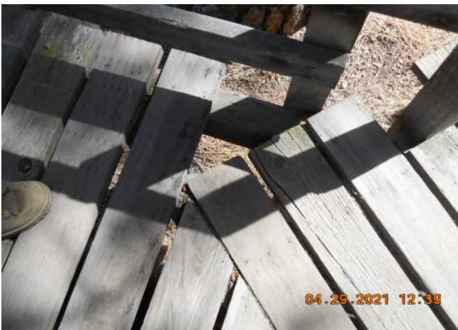
Deck Planking Not Full Width at Span 1 East End
