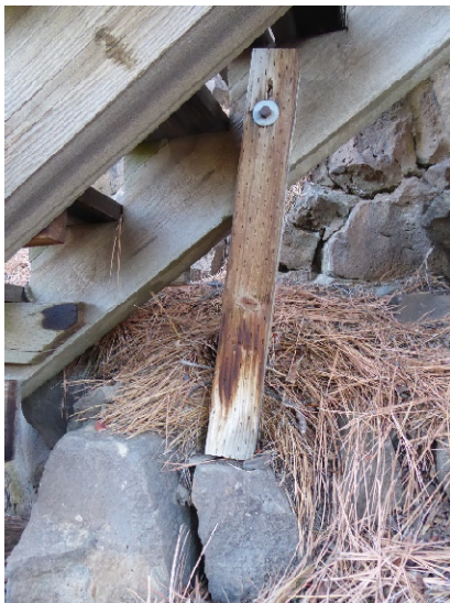
Photograph 6: Supports not positively connection to foundation.
