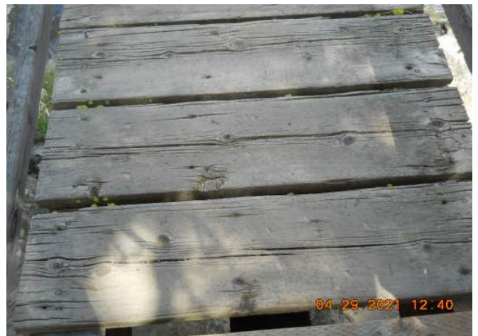
Deck Planking Splitting and Checking
