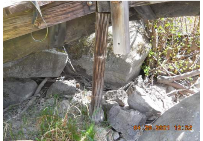
Bent 7 Post Floating
