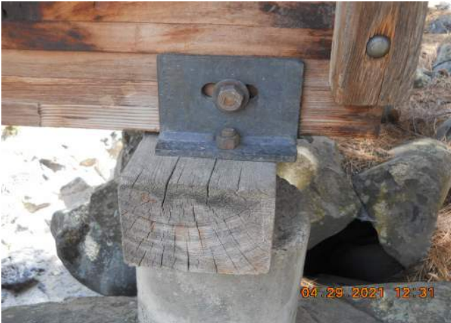
Bent 3 Bearing Plate Not Fully Bearing
