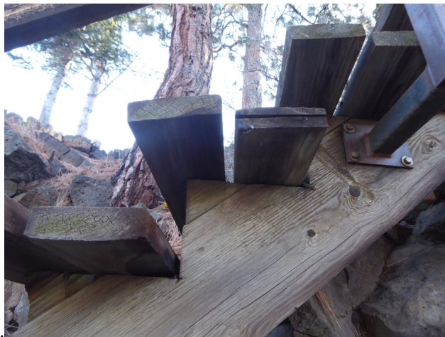
Photograph 4: Nosings not beveled and excessive overhang and gaps.
