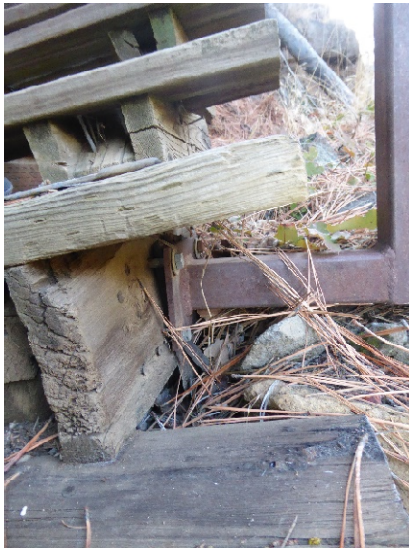
Photograph 7: Loose post connections.
