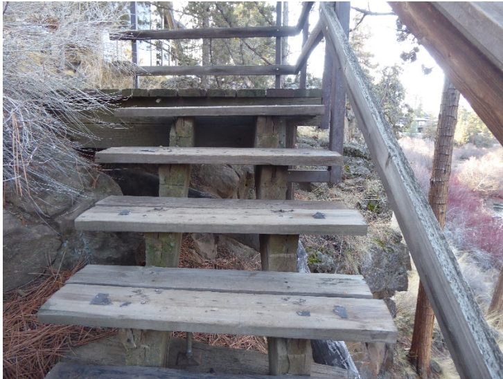
Photograph 3: Top riser not the same as height as others.
