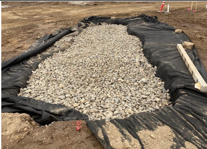
EXAMPLE OF ROCK INFILTRATION GALLERY UNDER CONSTRUCTION WITH GEOFABRIC
