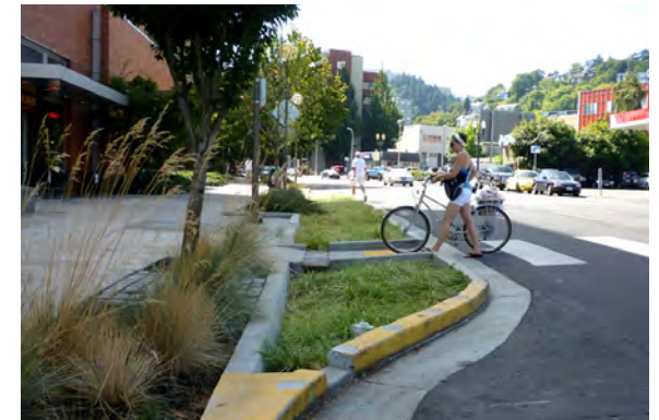
Mid-block crossing, curb extensions, stormwater treatment
