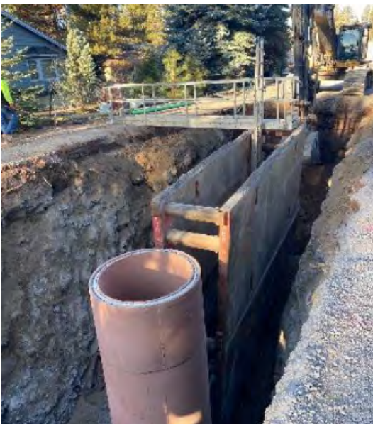
Manhole and pipe install
