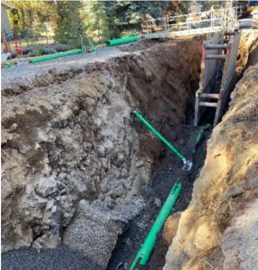
Eight-inch sewer and service lateral
