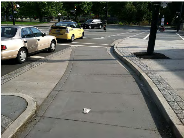
This photo shows the transition from separated to adjacent bike lane at the approach to an intersection.
