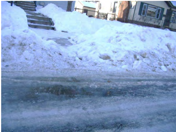
Slush gathers and refreezes on traditional asphalt whereas porous asphalt leads to slush free pavement: Case Study (photos taken January 17, 2010), Permeable Pavements in Cold Climates , John Gulliver, 2015.
