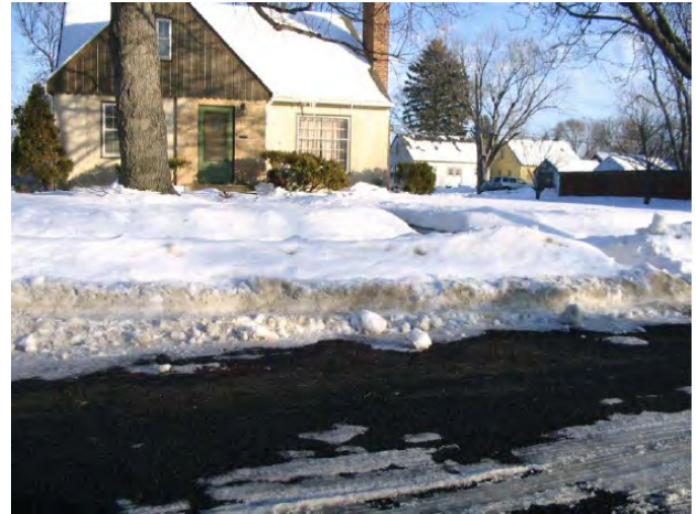
Slush gathers and refreezes on traditional asphalt whereas porous asphalt leads to slush free pavement: Case Study (photos taken January 17, 2010), Permeable Pavements in Cold Climates , John Gulliver, 2015.
