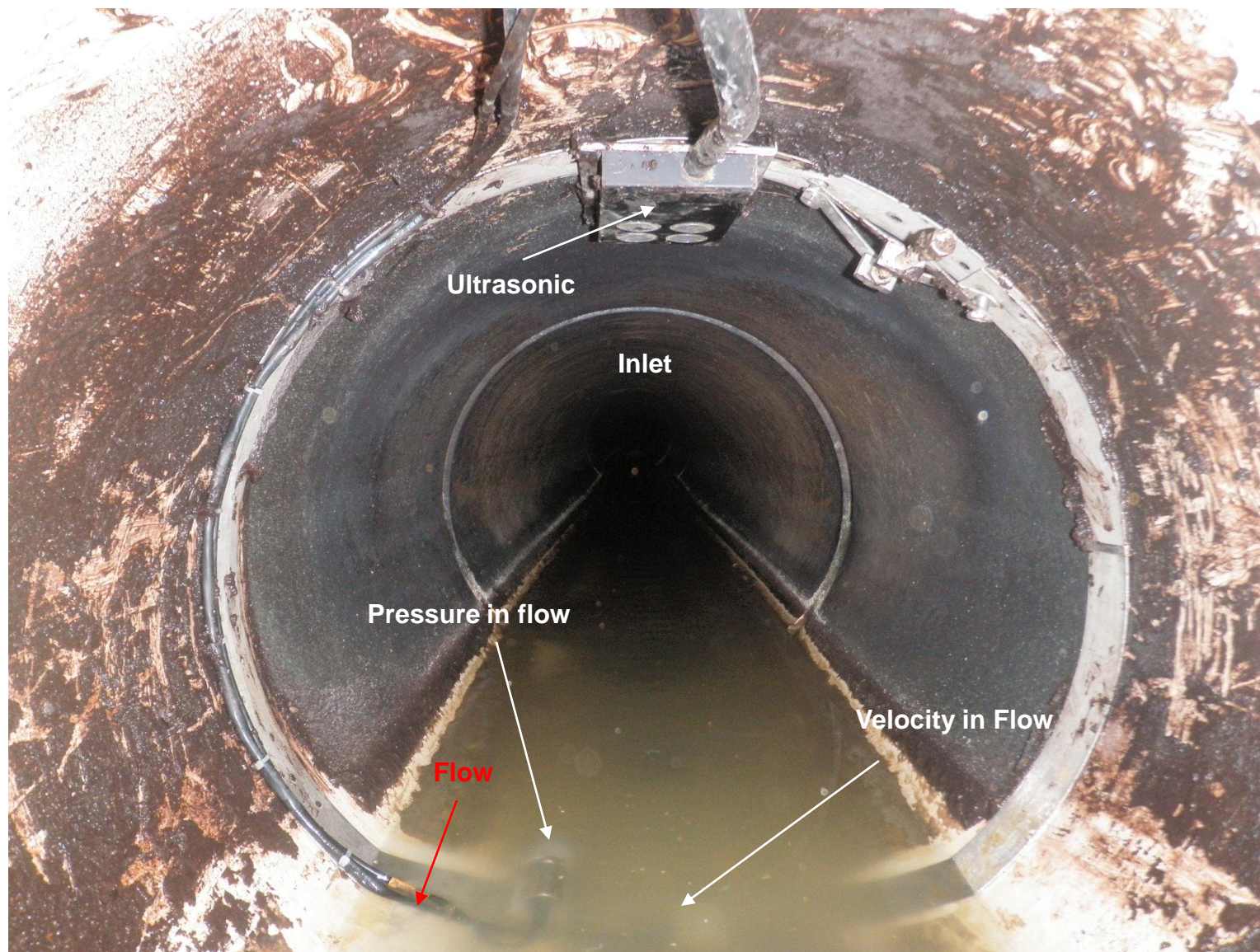
View of inlet and sensors
