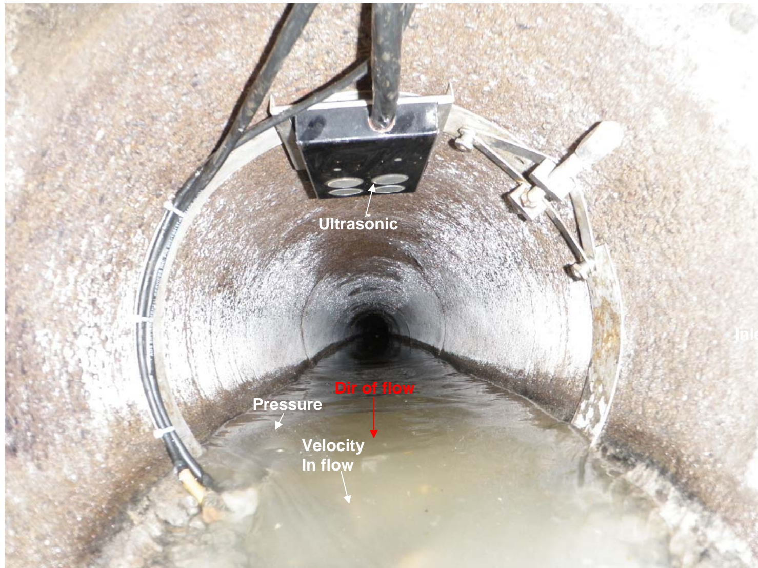
View of inlet and sensors
