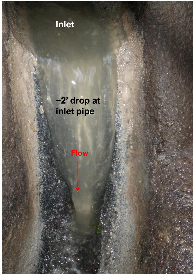
View of inlet and hydraulics
