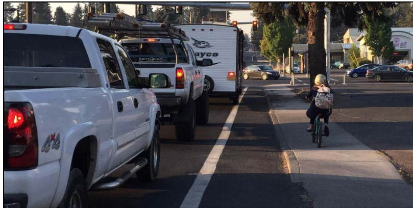
Figure 6 The basic bike lane on NE 8th Street is high-stress because it is on a 35 mph roadway and is narrow
