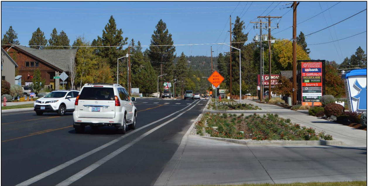
Figure 7 In 2018, the City reconstructed NW 14th Street in Bend to provide separated bikeways. The new design incorporated buffered bike lanes and wide sidewalks
