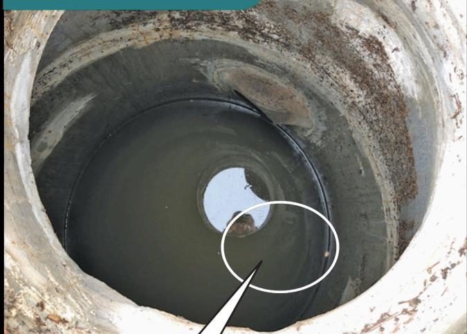
Perpetual stagnant water indicates that drywell has failed and needs to be thoroughly clean or replaced.
