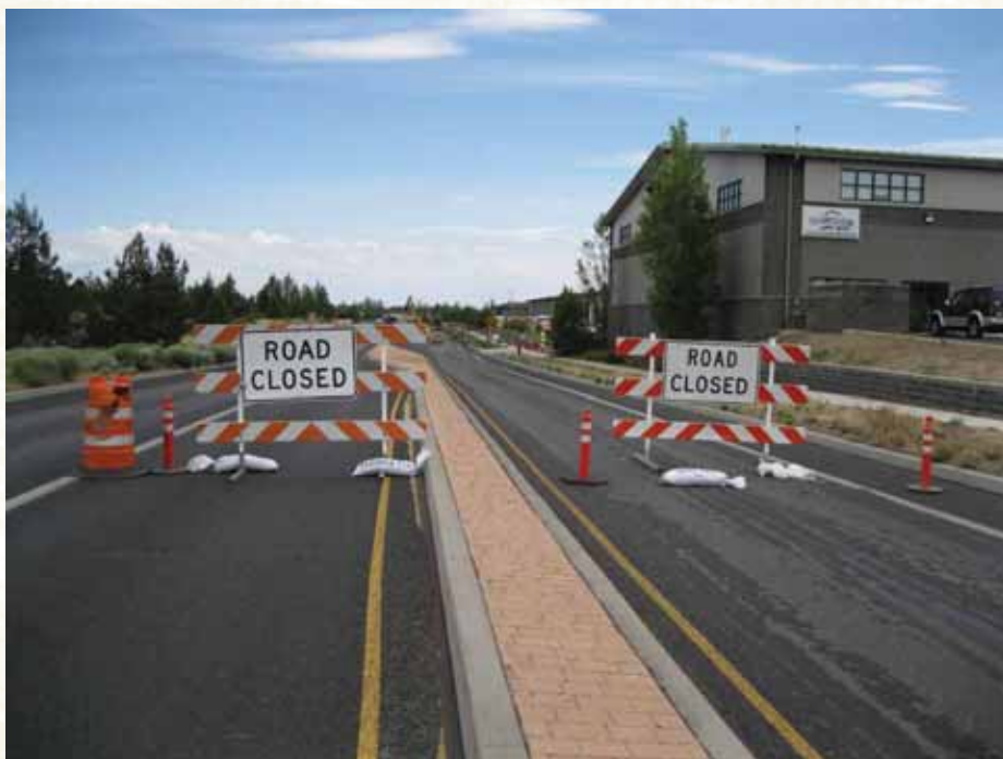
Construction - staged detour or segmented road closure.
