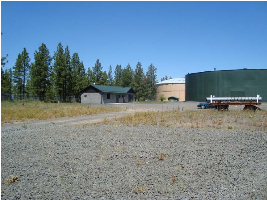
Figure 4 - North View of Existing Water Storage Tanks (proposed site in foreground)
