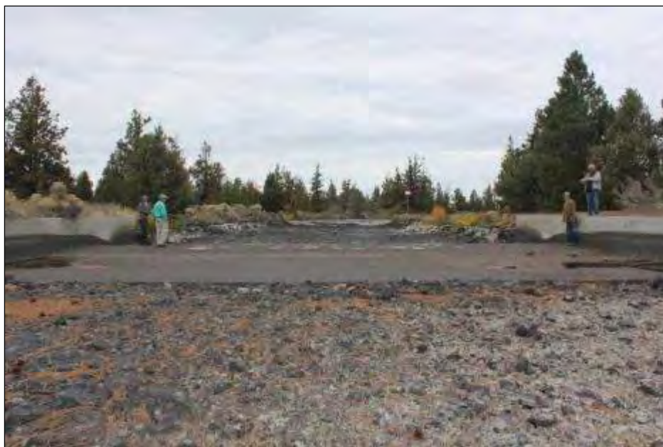
SEGMENT 5: The canal bed at its northern end is nearly flat and is wide and shallow. The surveyors are standing beside and in the 2012 concrete trapezoidal flow-measuring weir structure that was constructed in the existing canal bed. Photo looking north.
