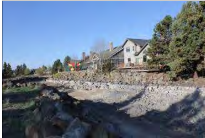
Photo shows altered riprap and extended embankment above waterline in Stretch 4, immediately south of historic district. Photographer looking southwest,
