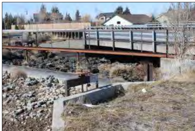
Photo shows some of the alterations to the canal in Stretch 4, immediately south of historic district: the new gate to a piped A-4 Lateral, a low head check, and a bridge at Empire Avenue. The bed under the bridge has been paved to prevent erosion. Photographer looking northwest.
