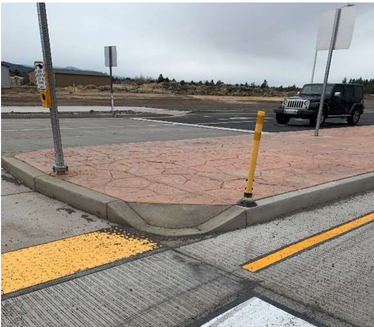
Figure 32. A beveled curb edge to facilitate snow plowing and prevent damage to curbs.
