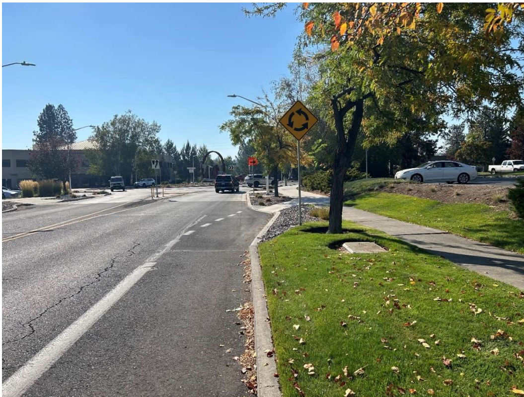
Figure 20. The curb in this photo is a great example of how to ensure decisive decision making by the bike rider. The curb clearly indicates that the lane is ending, and a choice must be made. (Southbound Columbia at Colorado)
