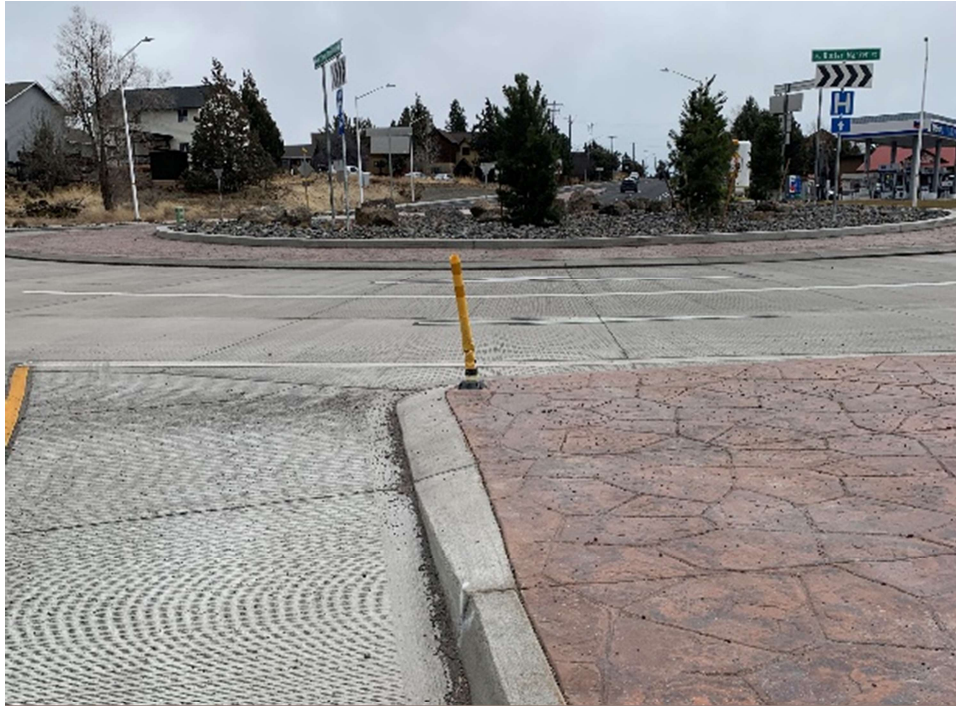
Figure A-5. This photo shows the use of mountable curb at the nose of a splitter island to facilitate use by larger vehicles that may need to use the splitter for turning movements and to facilitate snow plowing up to the edge of the circulatory.
