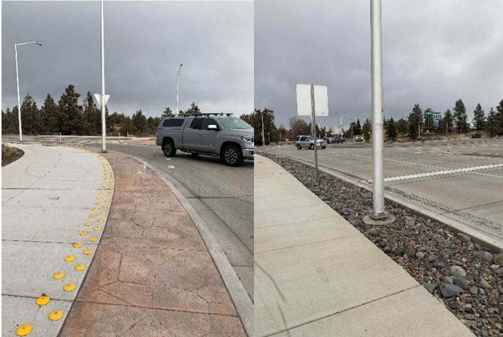
Figure A-3. PROWAG requires separation between the shared-use path around a roundabout and the road. The stamped concrete buffer did not provide adequate detectability, so the yellow detectable buttons were added to enhance its conspicuity. However this is not a preferred solution. The image on the right shows the use of decorative rock mulch, which is readily detectable.
