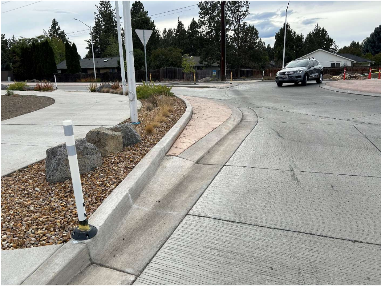
Figure 12. Curb-return mountable truck apron at the intersection of 15 th St. and Wilson Ave. This treatment allows for larger trucks to navigate a smaller ICD roundabout while maintaining speeds for everyday users.
