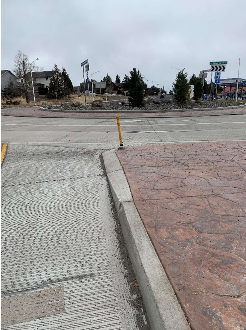
Figure 16. Mountable curbing on the splitter island corners adjacent to the circulatory roadway facilitate plowing and accommodates occasional oversize vehicles.
