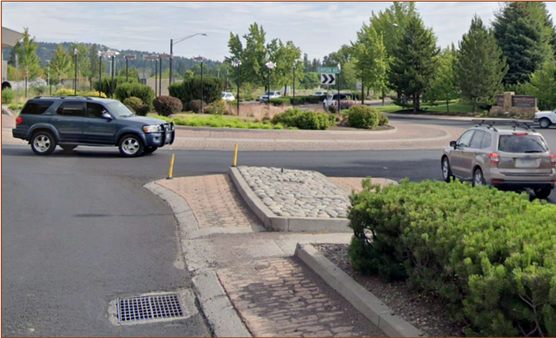
Figure 11. Double central truck aprons and stacked mountable/standard curbs allow for OSOW movements while maintaining a compact footprint. Intersection of Colorado Ave. and Simpson Ave.
