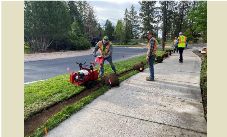
Sod removal with a motorized sod cutter and rolled sod strips.
