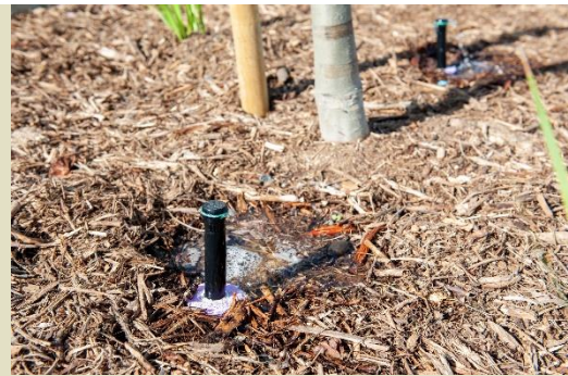
Tree irrigation to an established tree with multiple rings of inline drip tubing (left) and bubbler nozzles (right).
