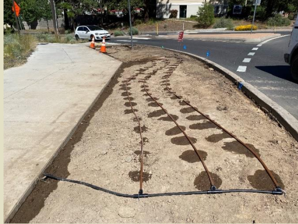
Inline drip irrigation- grid installation example demonstrating the uniform water application every 12".
