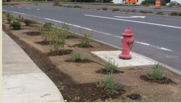
Point source drip irrigation- example demonstrating water application to individual plantings.
