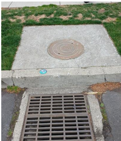
Stormwater manholes: curb intake and street intake
