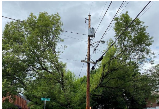
High Voltage: Tree pruned away from wires Telecoms: Not pruned from wires
