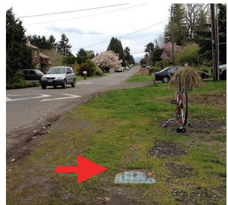
Clue: Water Meters at the edge of the ROW
