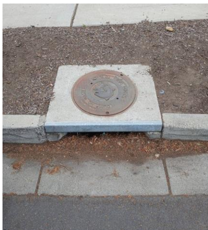
Stormwater manholes: curb intake and street intake
