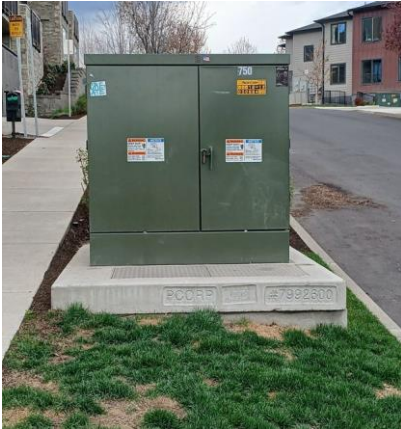
Electrical transformer
