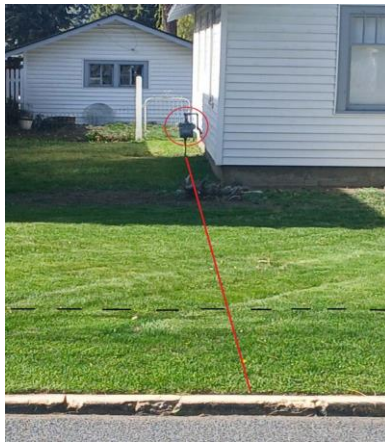
Gas lines coming from house mounted meters
