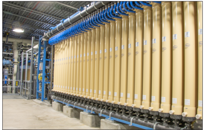
Above: Bridge Creek Water Intake, winter 1948. Below: Membrane filtration system at Outback Water Filtration Facility.
