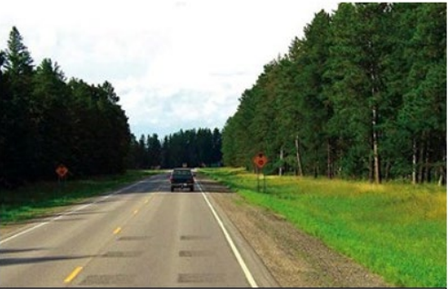
Rumble Strips Before Intersections (Potential Crash Reduction = 25%)
