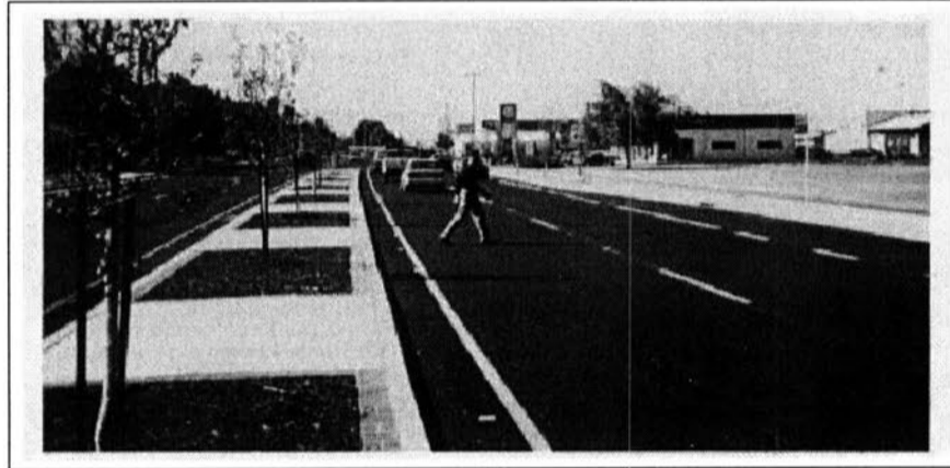
Figure 22. Median allows pedestrian to cross one direction of traffic at a time Source: Oregon Bicycle & Pedestrian Program
