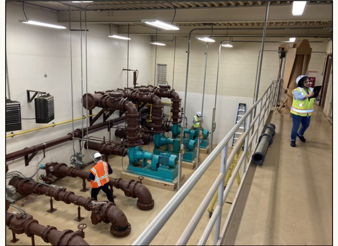
Pictured: Carollo Condition Assessment Team reviewing RAS/WAS Pump Station
