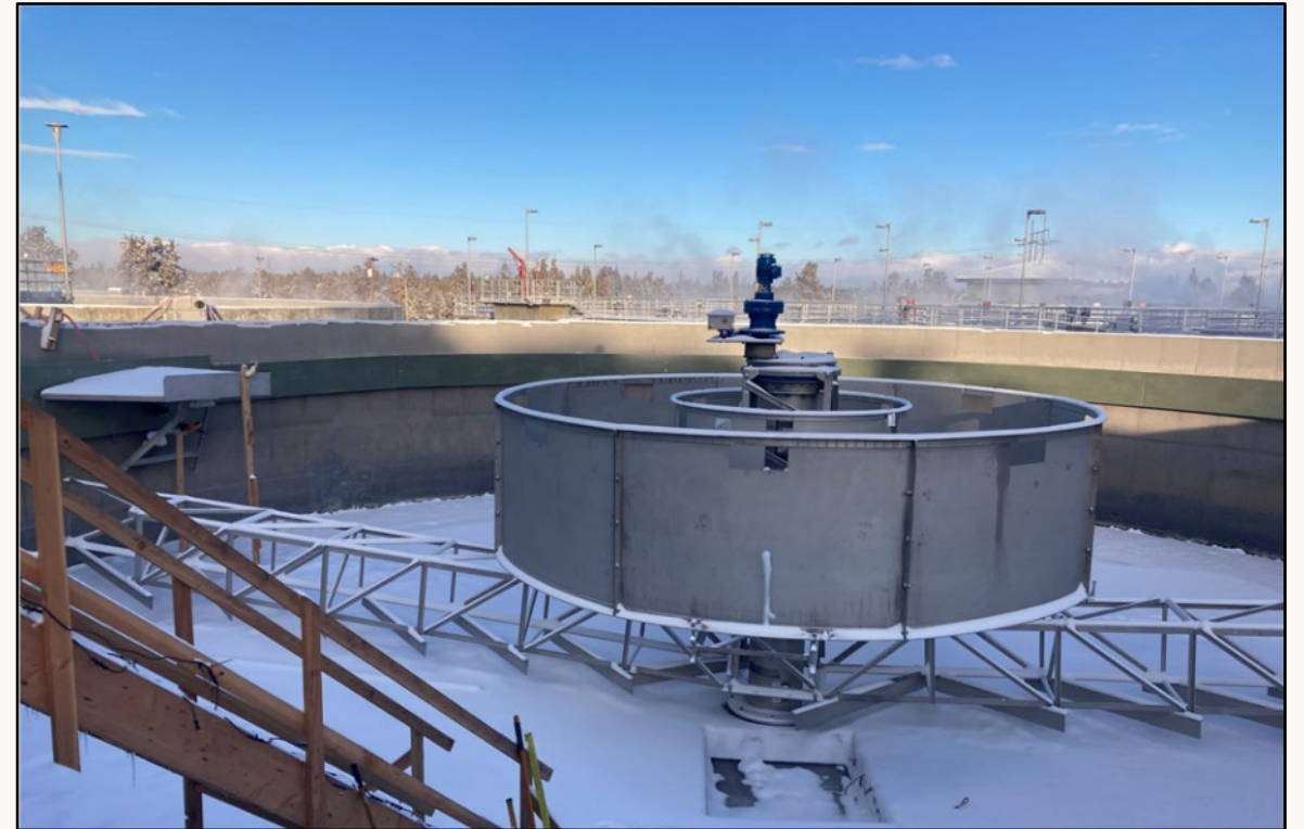
Pictured: Primary Clarifier No. 1 Improvement Project (Previous R&R Project)
