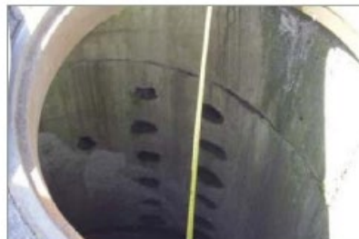
Figure 1-1. Drill hole (top); drywell interior (bottom)
